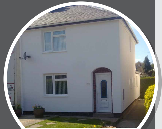
House with external wall insulation
